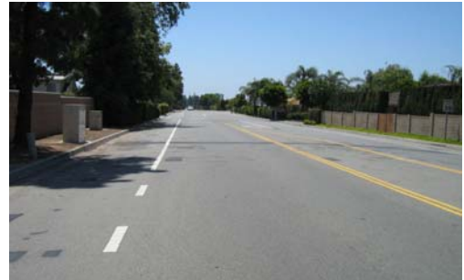
Taft Avenue Landscaped Medians Improvement Location
