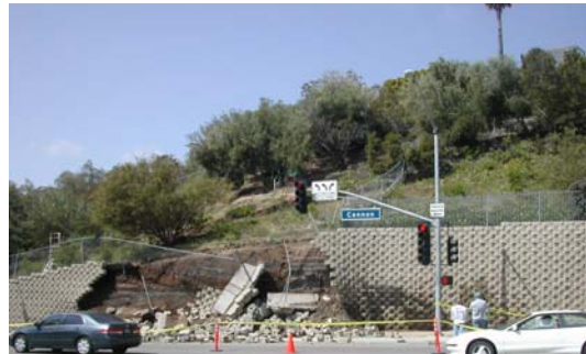
Cannon Street Retaining Wall Improvement Location
