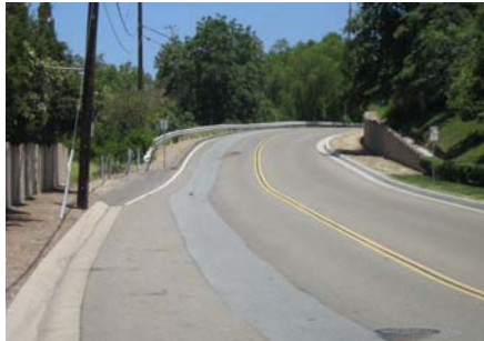
Mesa Street Guardrail Improvement Location
